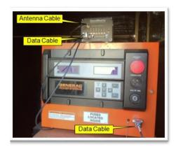
Data Cable and Antenna Cable Connections.
