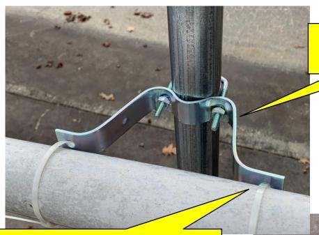
Attach the wall mounts to the mast
