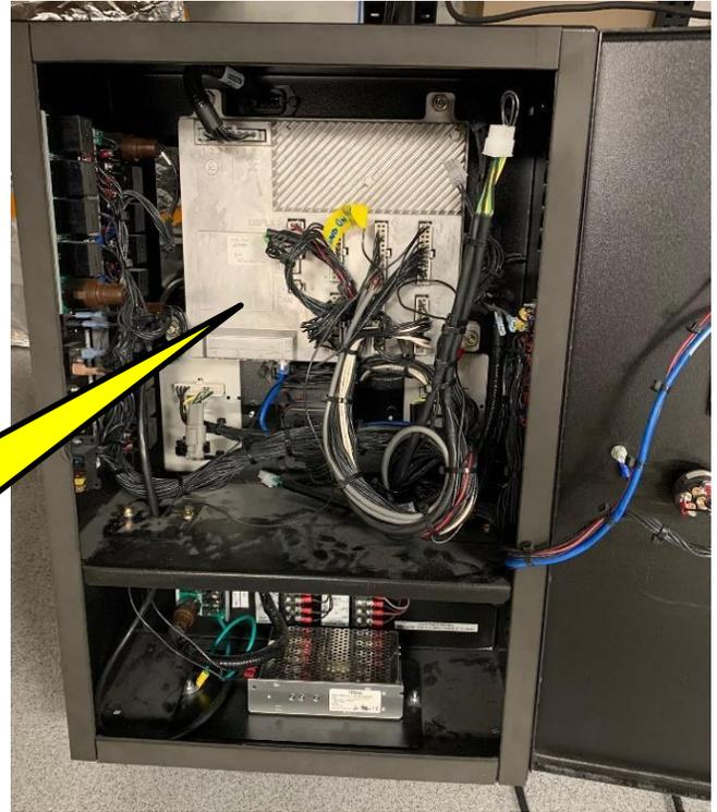
**For reference, this is the PowerZone Synch Control. No connection from the OmniMetrix monitor is made to this panel.**
