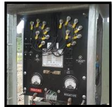
(Figure 2) Completed Installation
